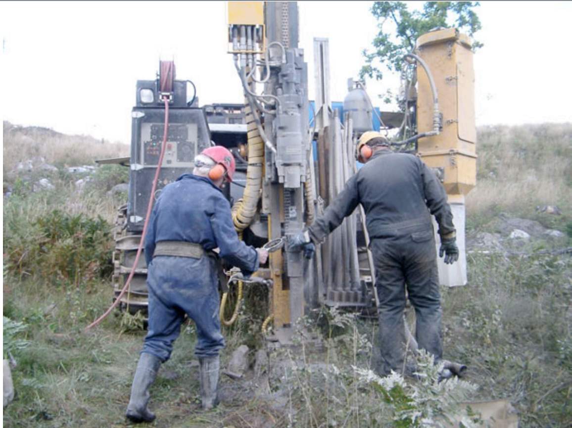
Shallow drilling at Grönhög
