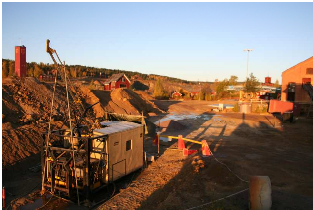
Photograph 2. Drill rig, Hole 11-09
