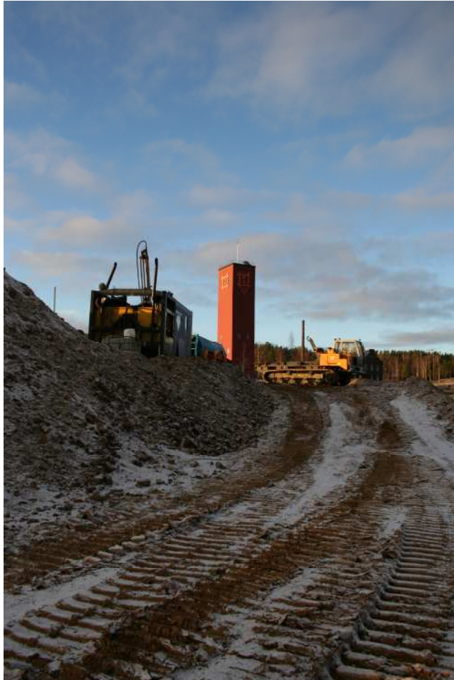
Photograph 3. Drilling of Hole 12-09 (hole currently being drilled)
