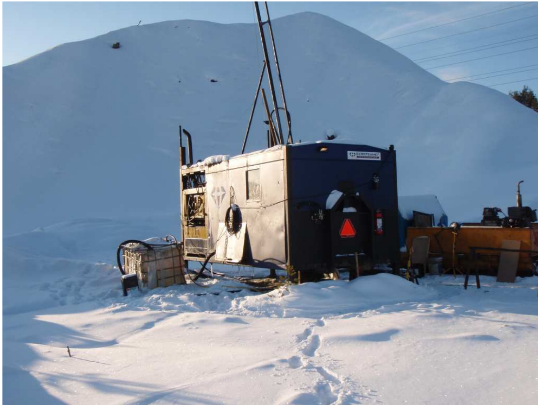
Drill rig on Site 18-10, March 2010
