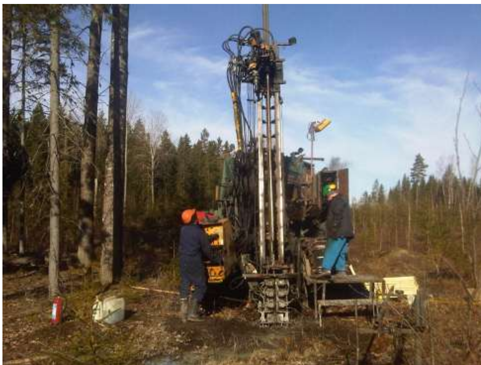
Drilling at 12DDTS003, March 2012
